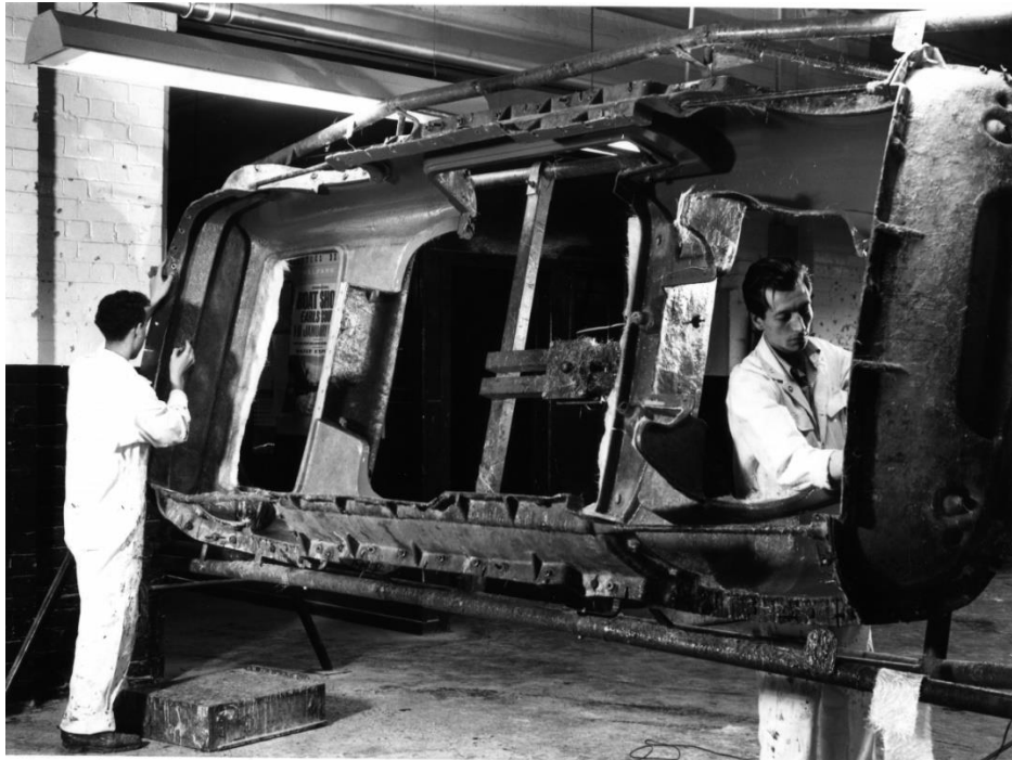
An Elan 1500 body being constructed on a rotisserie at Bourne's Nottingham works
